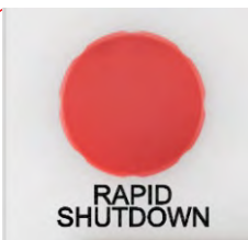
Figure 5.15 Inverter rapid shutdown and EPO initiation switch
